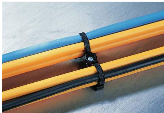
Parallel fixing of two cables
